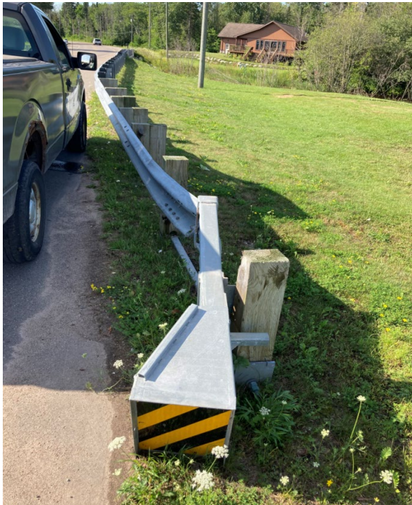
3: 1914 Riverside Drive: 12 feet W-Beam guard rail. Reinstall Fleet end section.
