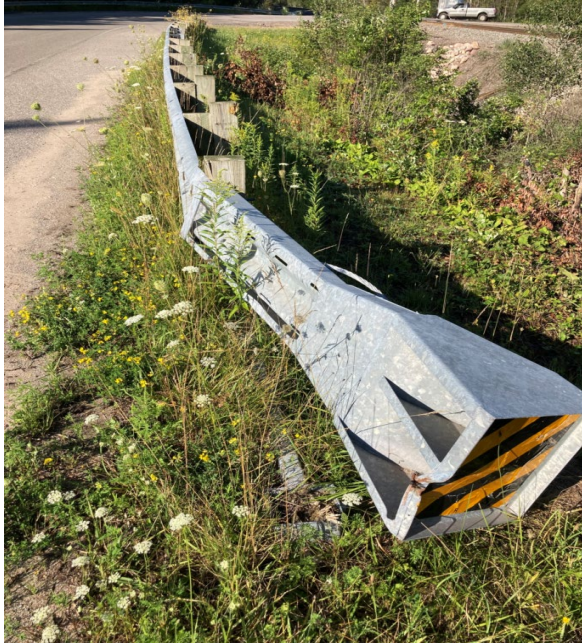
3: 1914 Riverside Drive: 12 feet W-Beam guard rail. Reinstall Fleet end section.
